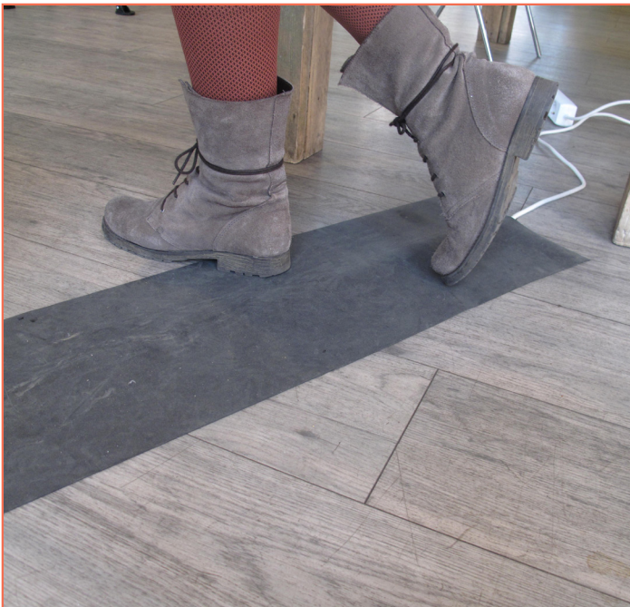
Safe: extension cords covered with rubber mats
